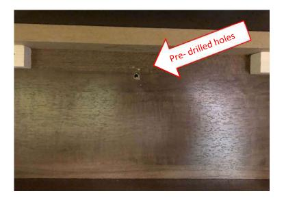
10.Place a screw in each of the holes – and tighten the screws with a Phillips head – power drill.
