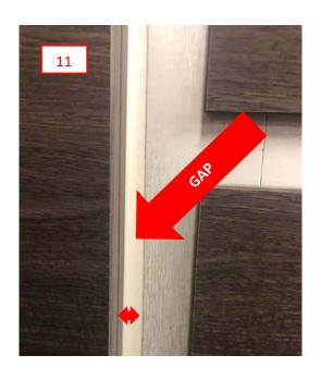
12.To complete the placement process – simply adjust the *Wall Guard* to close the gap – and run a screw through the *Bottom Cleat* – into the predetermined wall stud
