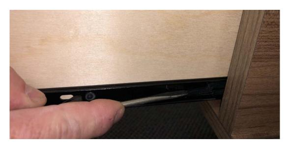
6. **LEFT SIDE** - Place a flat tip screw driver into the gap between the cabinet side and drawer side – and move the lever upward. *When the lever moves - pull the left side of the drawer out slightly.*
