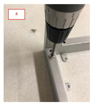
4. Using the *4mm Hex Insert*– drive the *Hex Bolts*tightly into place.
